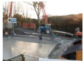
New foundation for future house
