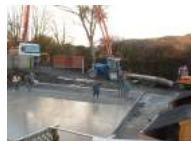
New foundation for future house
